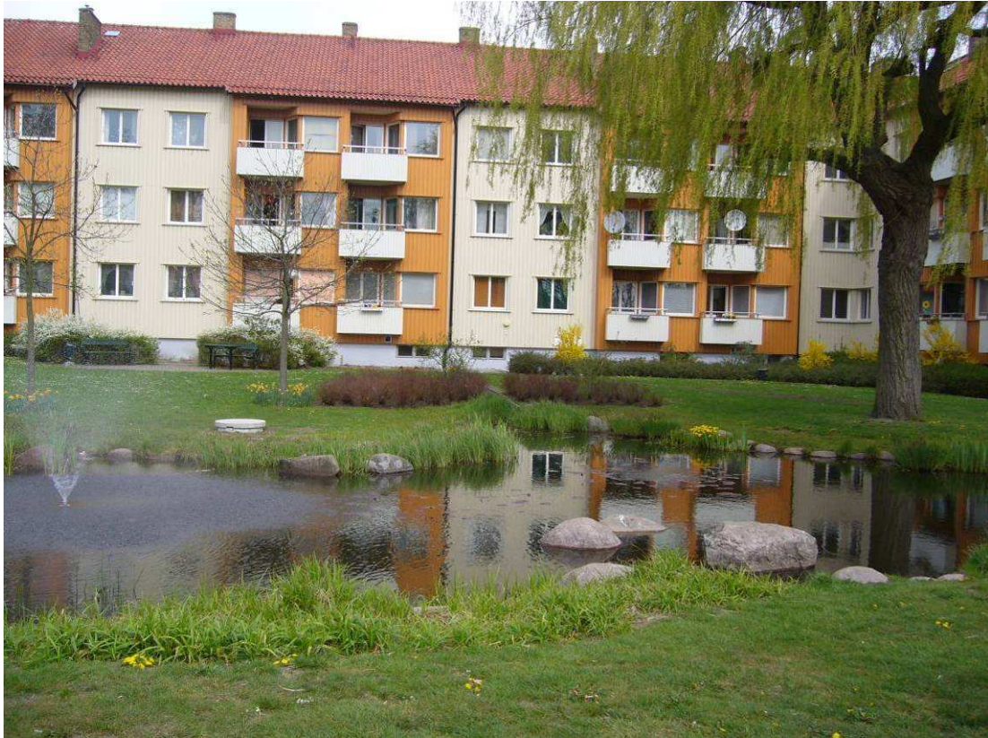
Figure 2. Sustainable urban drainage system in Augustenborg (Photograph: GRaBS)
