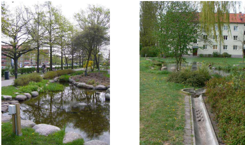
Figure 3. Sustainable urban drainage system in Augustenborg (Photograph: GRaBS)
